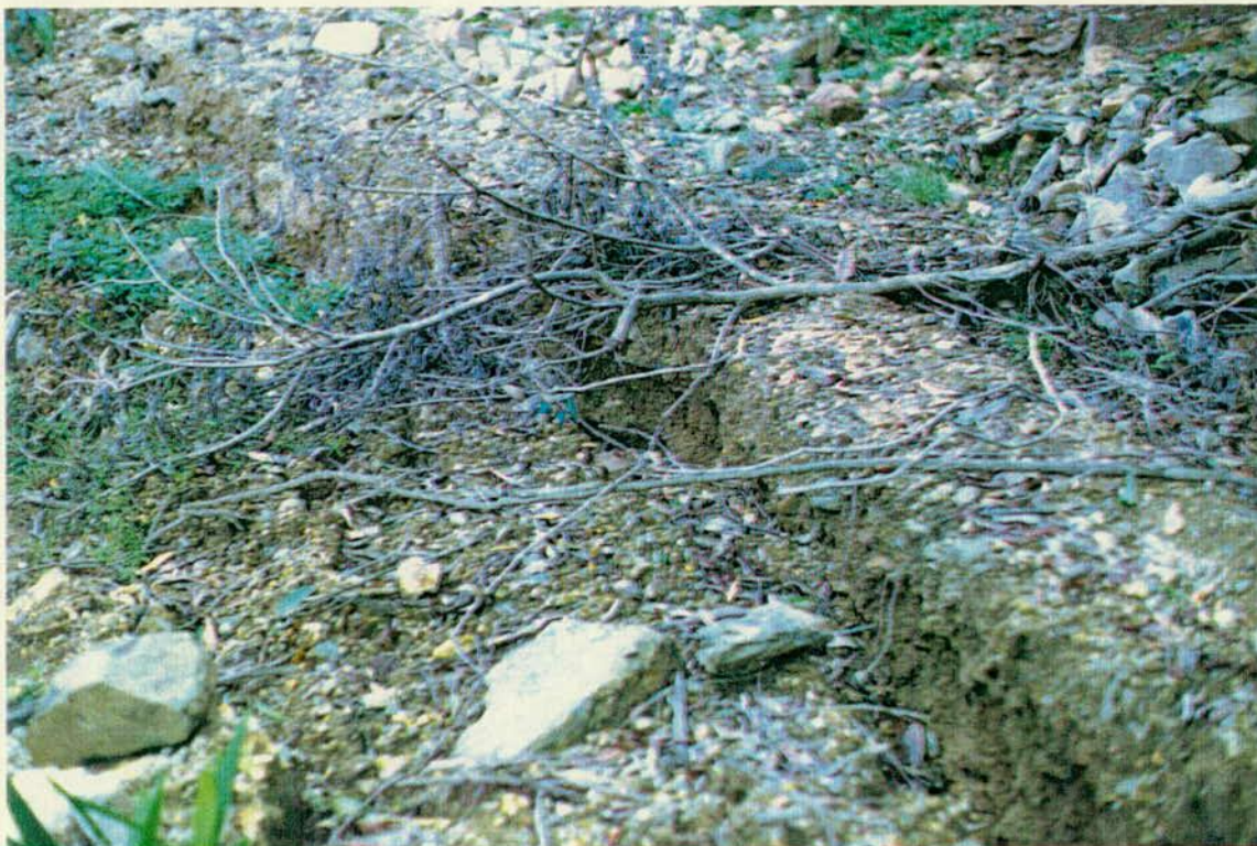
SLUMPS OF SNIG TRACK PAVEMENT.
