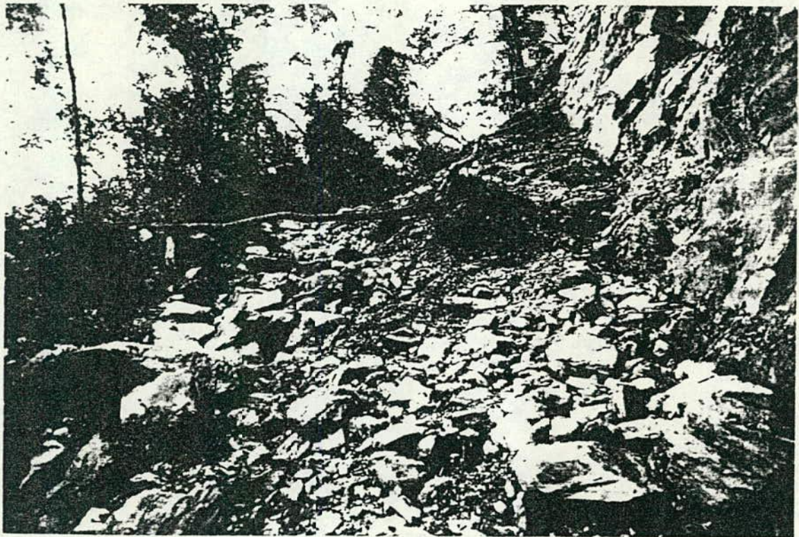
CUT BATTER FAILURE ON SNIG TRACK SC1
