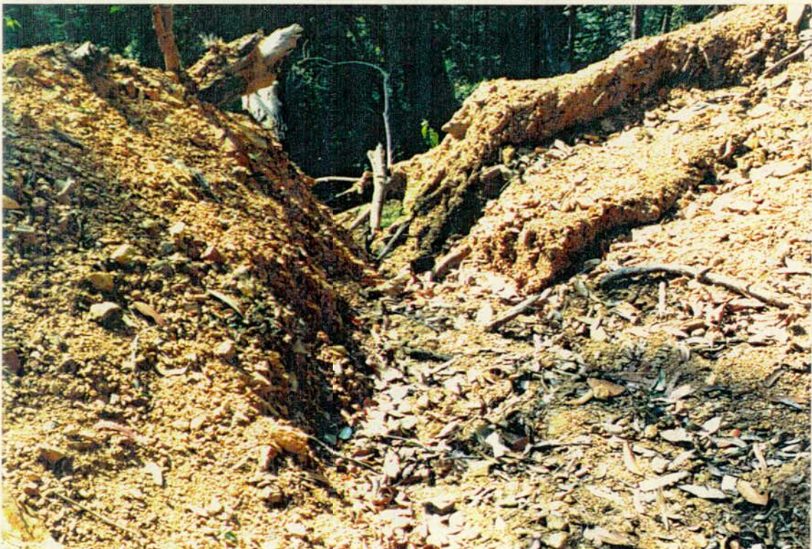
ERODED OUTLET ON CROSS BANK.
