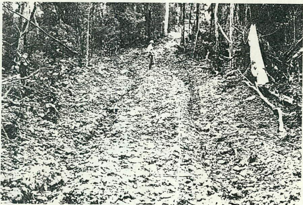
BOX CUT RIDGE TRACK SC5 HIGH WINDROWS RILLED DOWN DOZER TRACKS.
