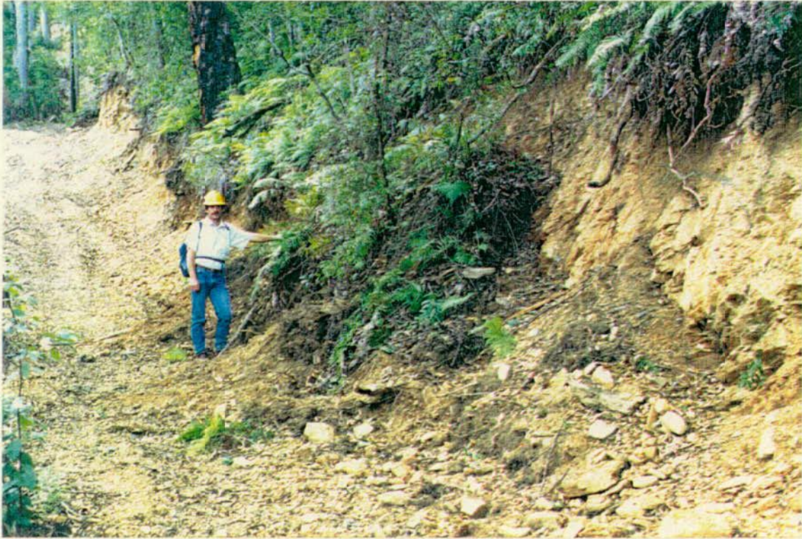
CUT BATTER FAILURE ON SNIG TRACK SC1
