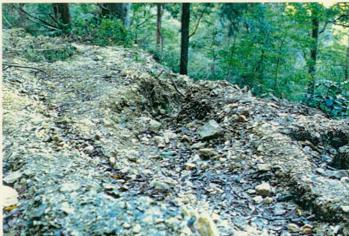
SLUMPS OF SNIG TRACK PAVEMENT.
