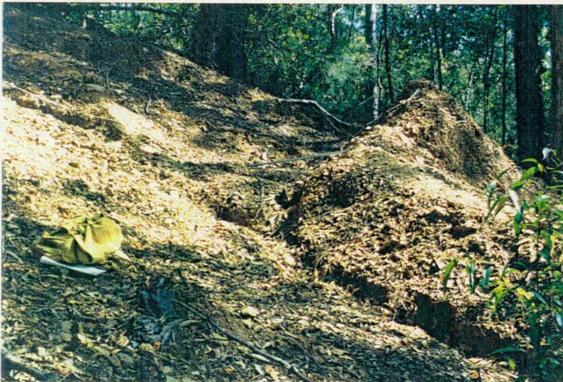
INEFFECTIVE BANK ON SIDECUT SNIG TRACK. RILLED DOWN TRACK AND THROUGH OUTLET.
