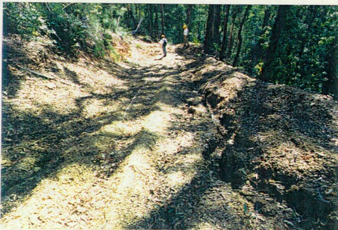
BOX CUT SIDECUT SNIG TRACK WITH HIGH WINDROW PREVENTING WATER EXIT. RILL ON WINDROW TOE.
