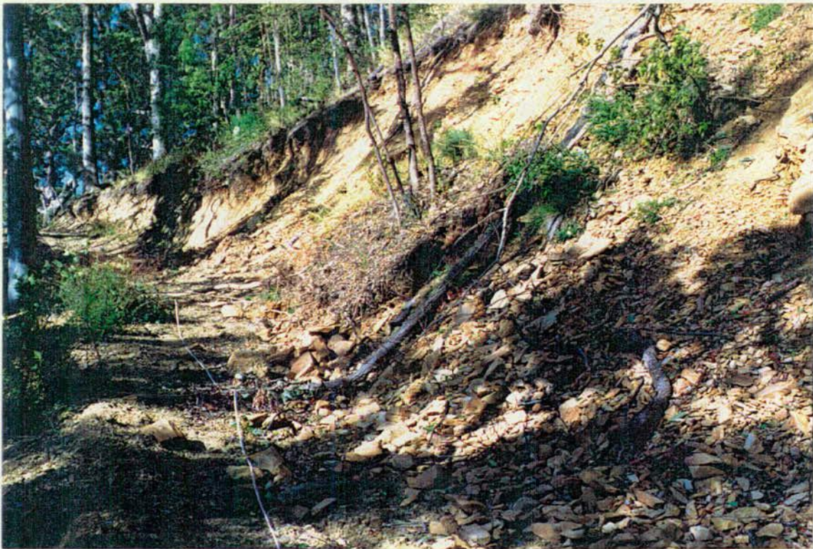
LARGE CUT BATTER AND SLIP ON SNIG TRACK SU6 FROM DUMP 7 UPSLOPE.
