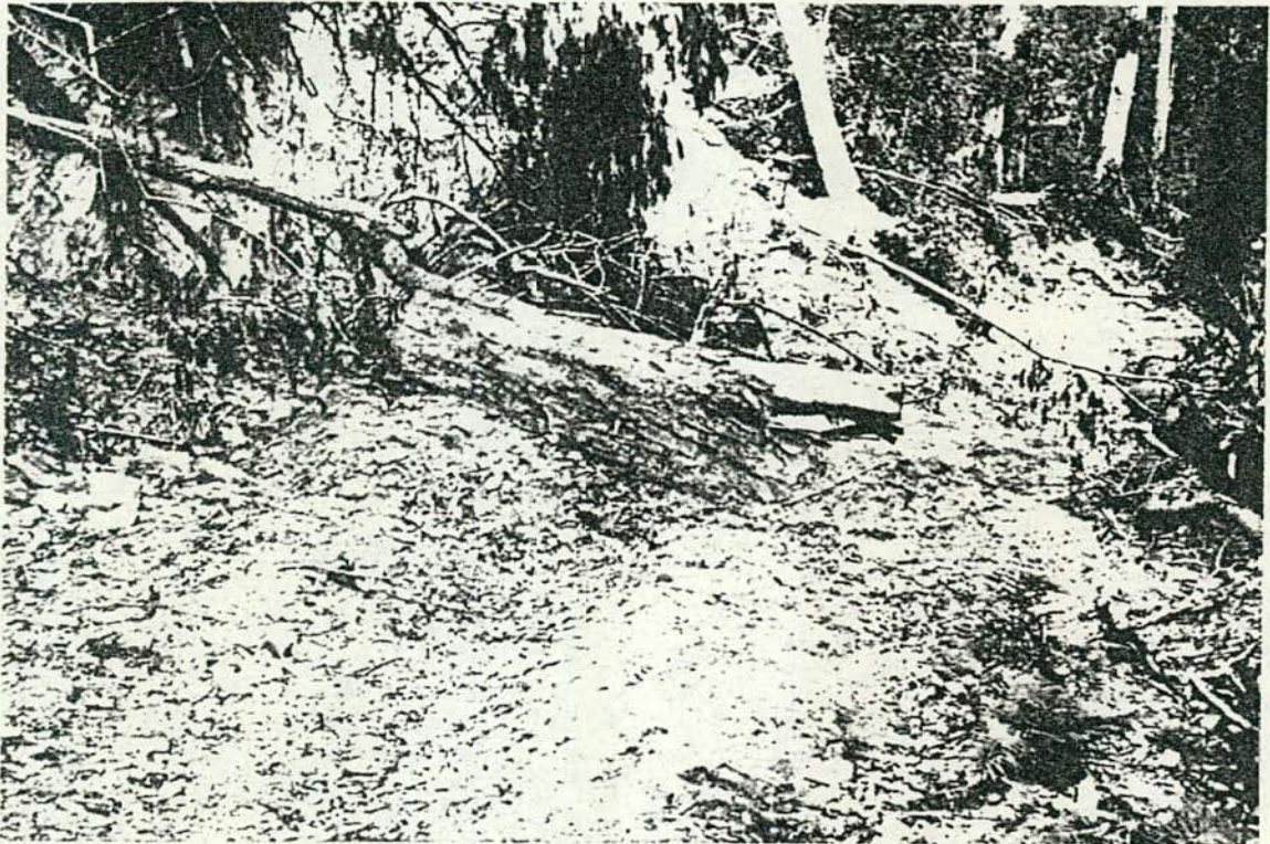
SIDECUT SNIG TRACK SU6 FROM DUMP 7 INEFFECTIVE BANK.
