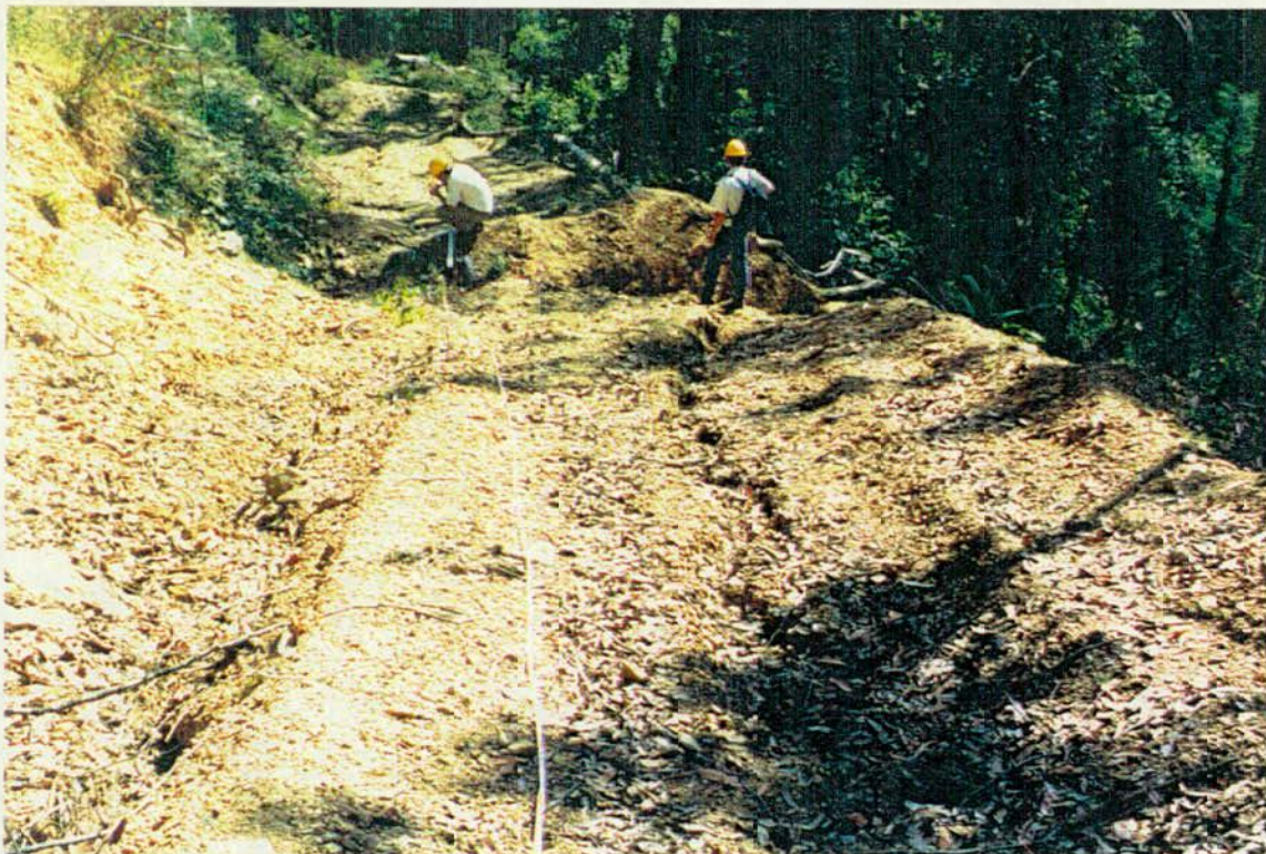
INEFFECTIVE BANK ON SIDECUT SNIG TRACK. RILLED DOWN TRACK AND THROUGH OUTLET.
