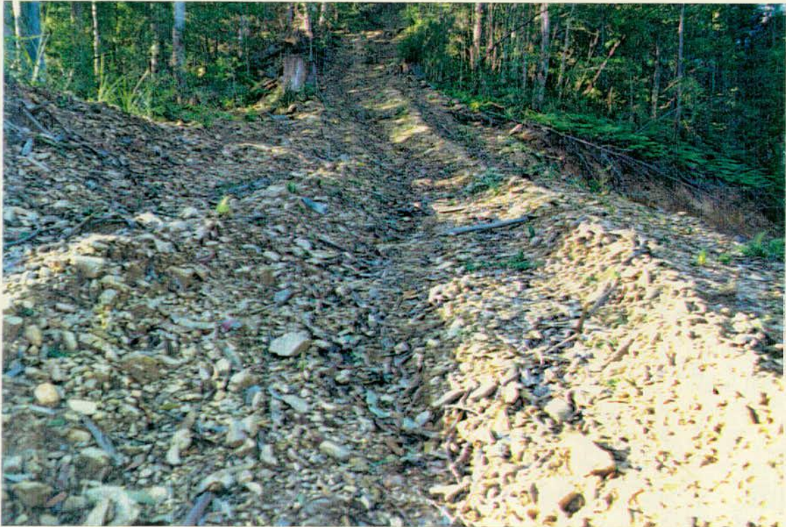
RIDGE SNIG TRACK WITH DEEP LOG SCOUR.
