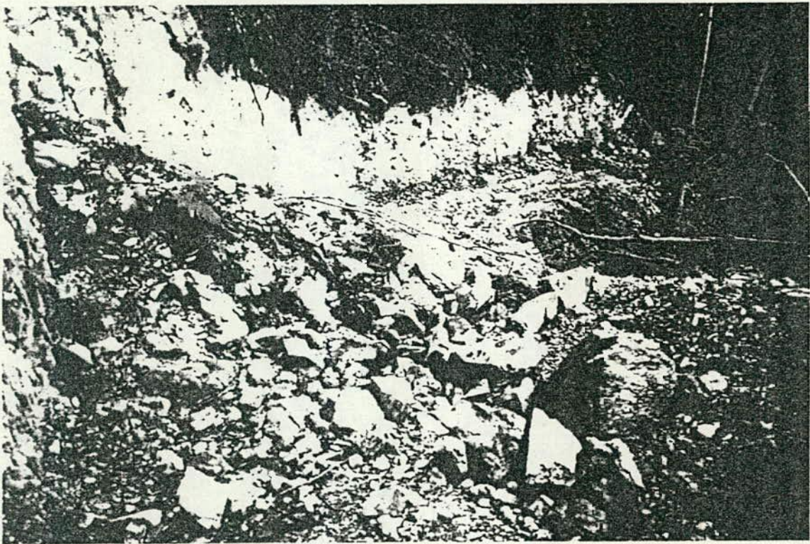
SLIP OF ROCK ON SNIG TRACK SUS FROM DUMP 5 DOWNSLOPE.
