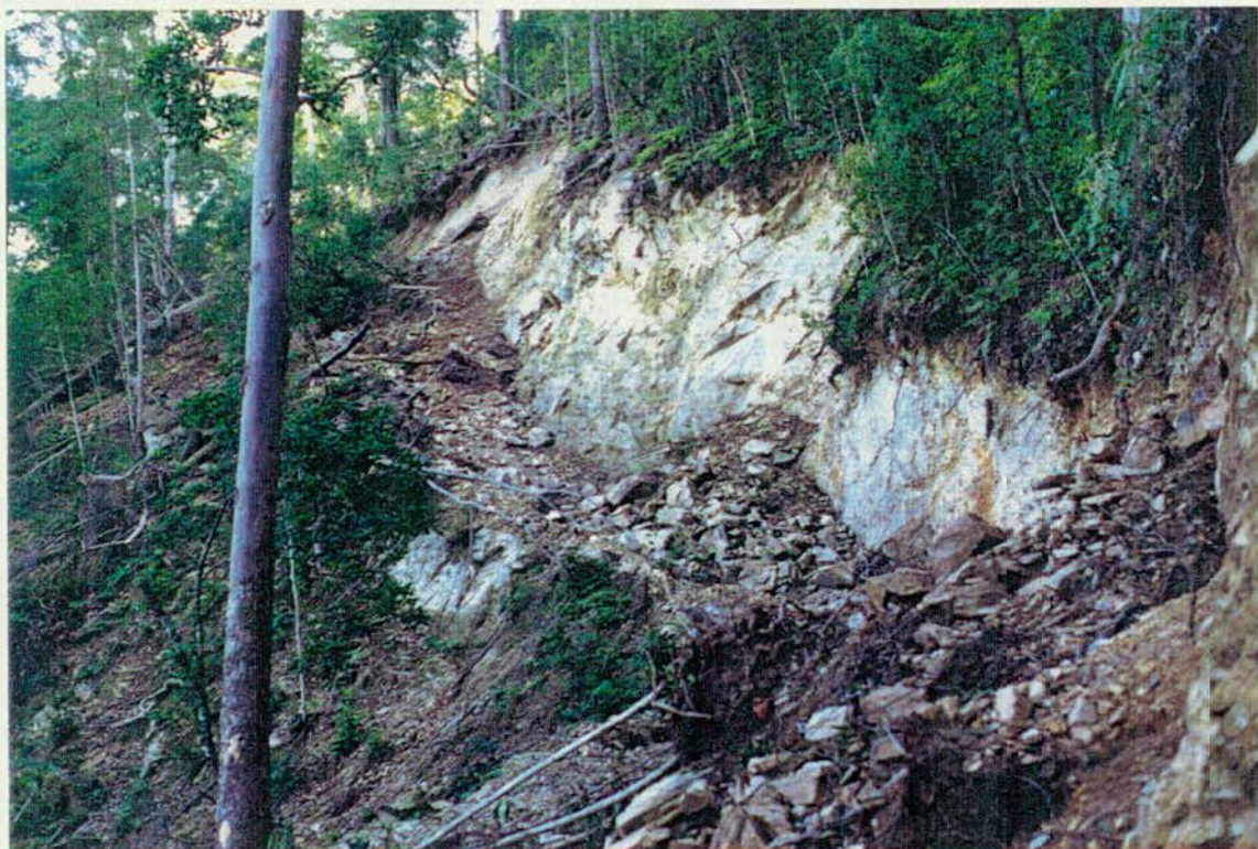
SLIP OF ROCK ON SNIG TRACK SU5 FROM DUMP 5 UPSLOPE.
