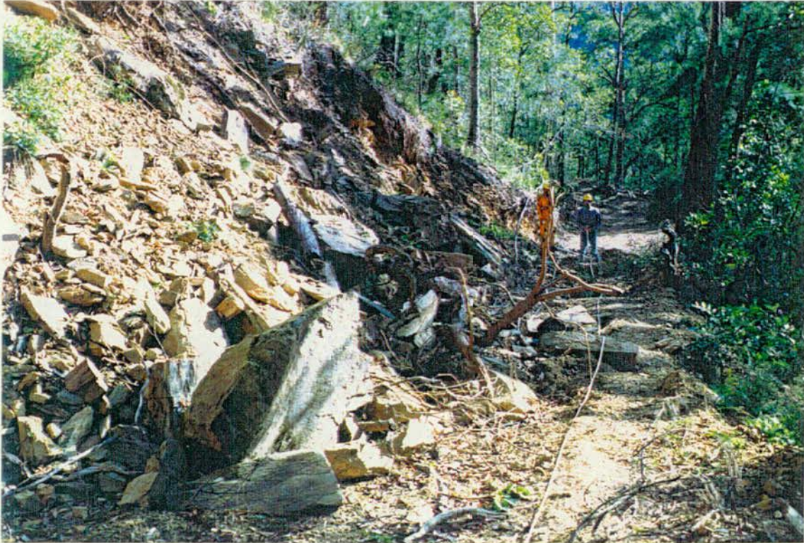
LARGE CUT BATTER AND SLIP ON SNIG TRACK SU6 FROM DUMP 7 DOWNSLOPE.
