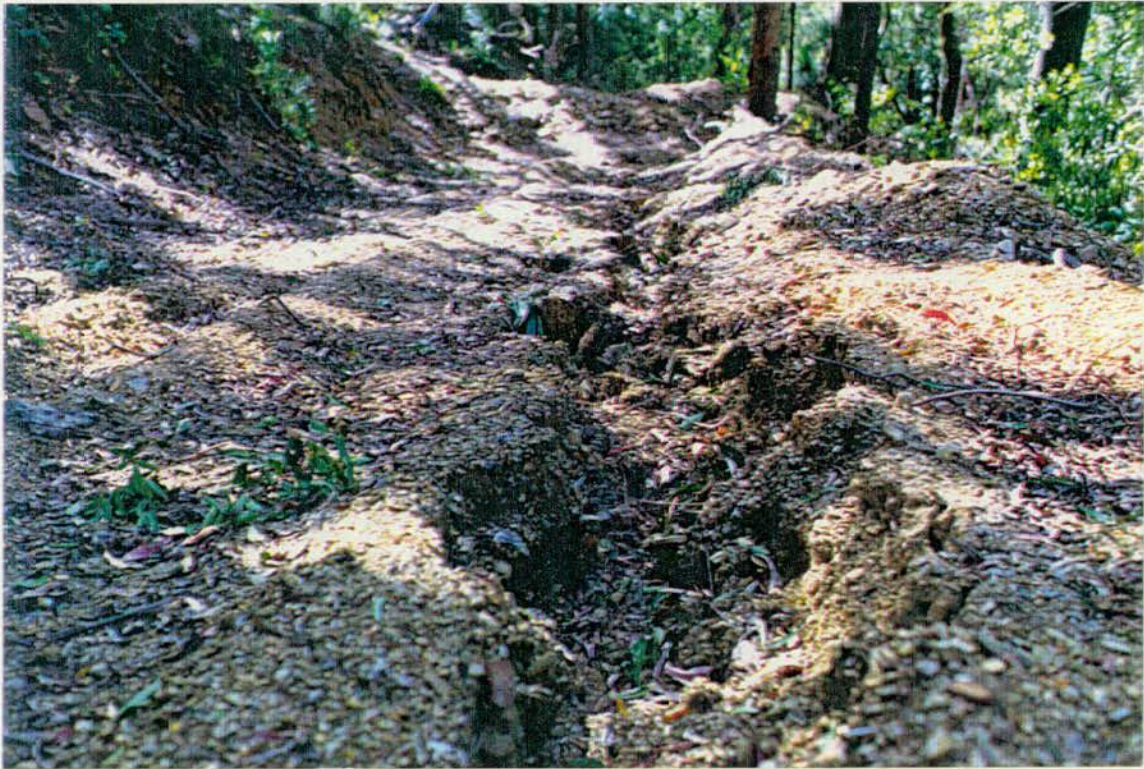
SIDECUT SNIGTRACK, UPSLOPE WITH HIGH WINDROW AND DEEP RILL
