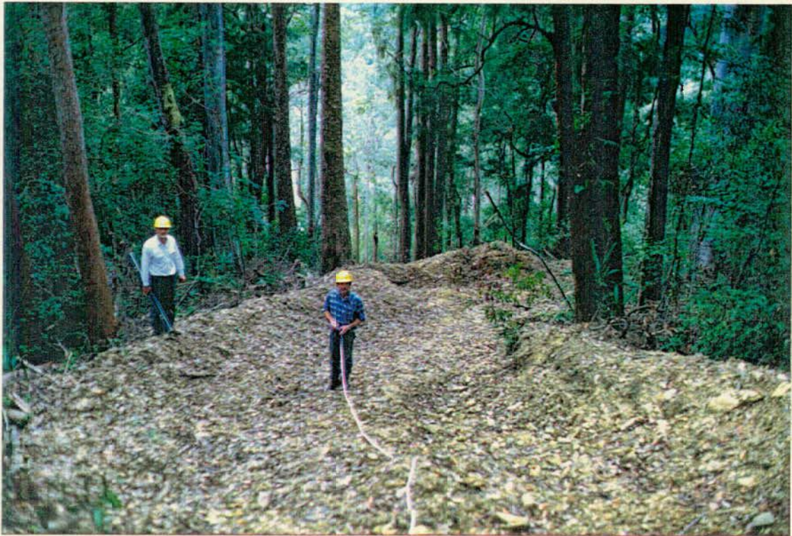
BOX CUT RIDGE TRACK SC5 HIGH WINDROWS AND RILLED.
