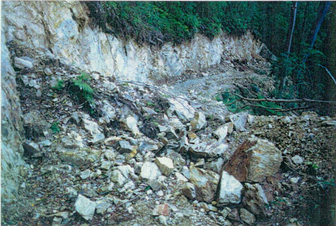
SLIP OF ROCK ON SNIG TRACK SU5 FROM DUMP 5 DOWNSLOPE.
