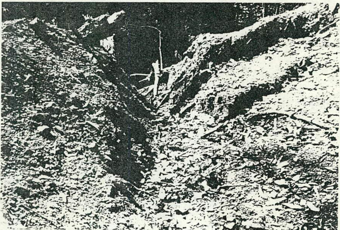
ERODED OUTLET ON CROSS BANK.
