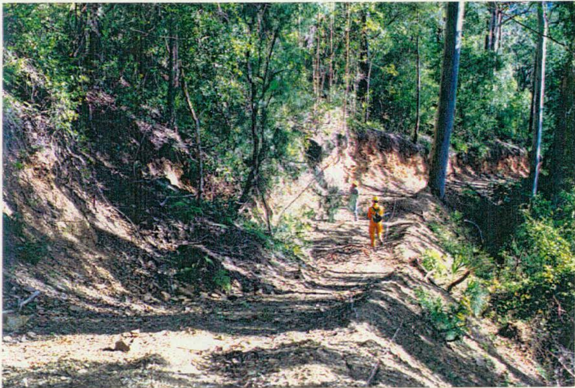
SLIP ON SNIG TRACK SU6 FROM DUMP 7 DOWNSLOPE. NOTE WINDROW
