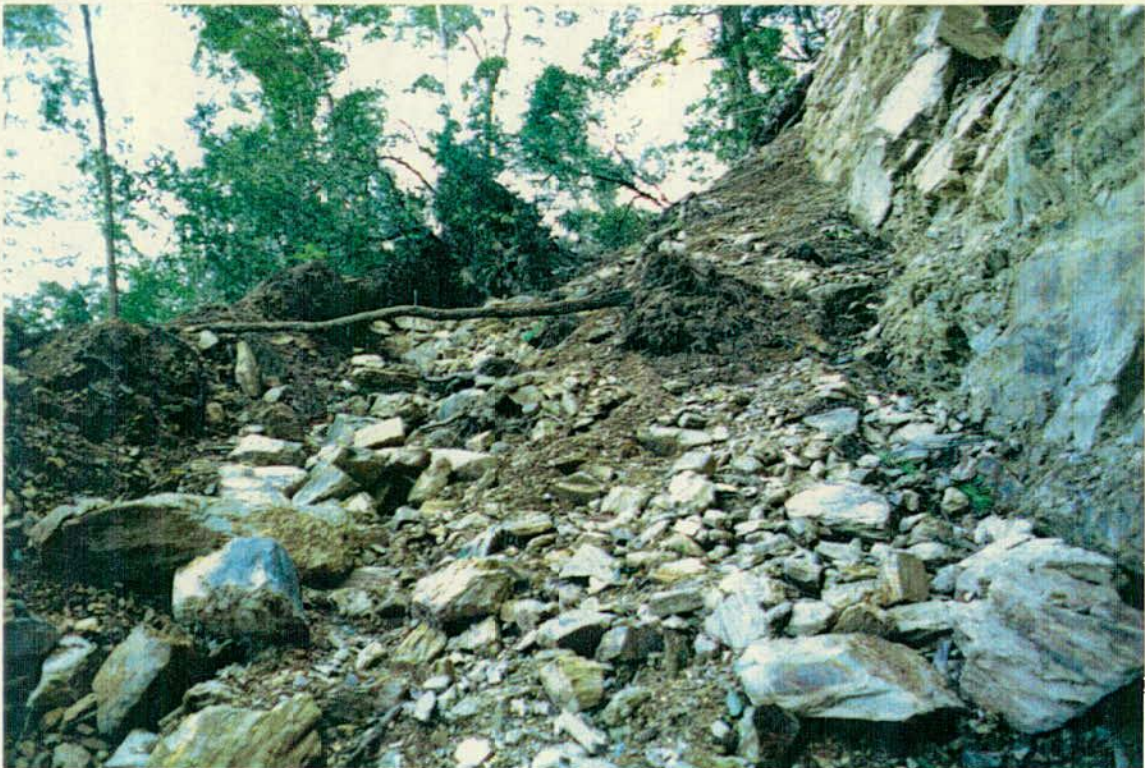
CUT BATTER FAILURE ON SNIG TRACK SC1
