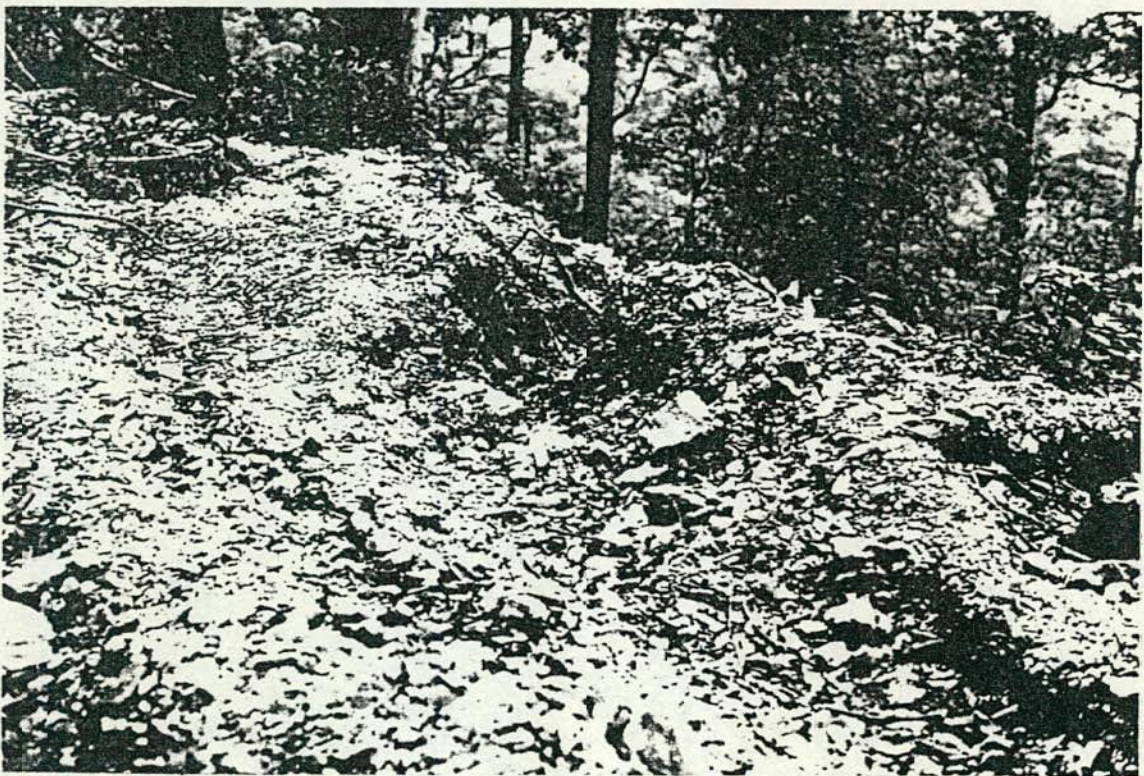
SLUMPS OF SNIG TRACK PAVEMENT.
