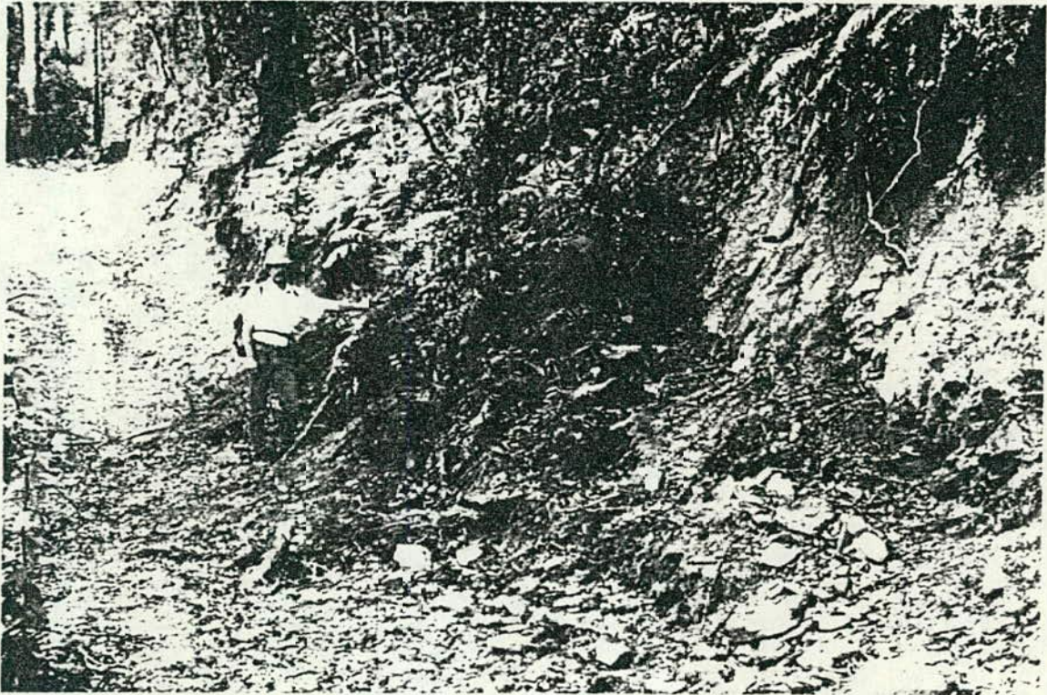
CUT BATTER FAILURE ON SNIG TRACK SC1
