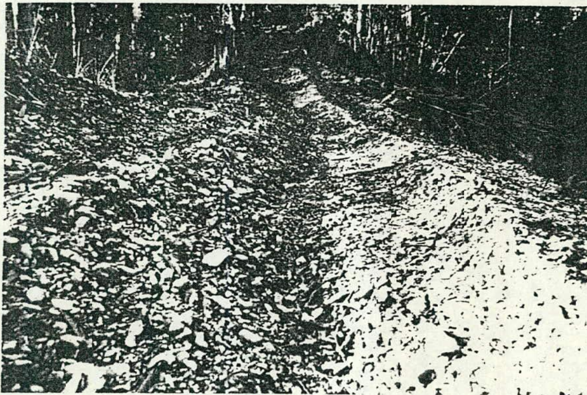
RIDGE SNIG TRACK WITH DEEP LOG SCOUR.
