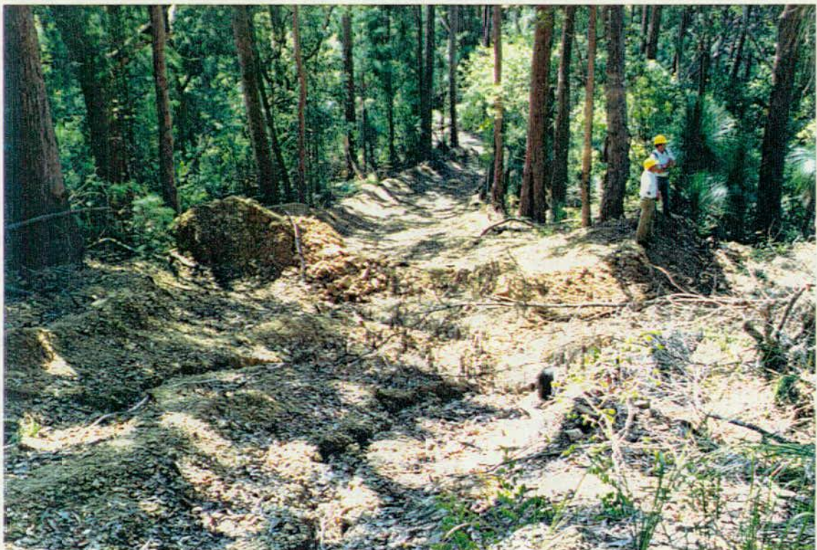
BOX CUT RIDGE LINE SNIG TRACK SC5 WITH INEFFECTIVE BANK. TRACK RILLS FOLLOWING RIGHT BRANCH TRACK.
