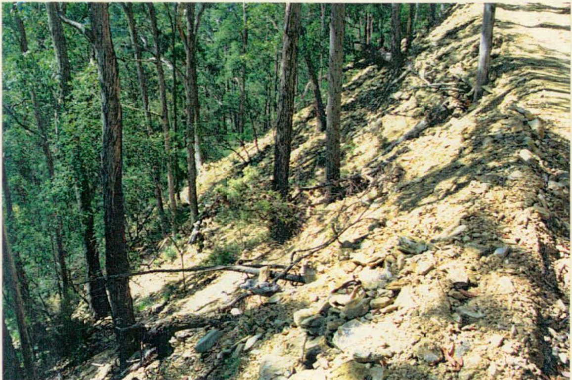
CATBIRD ROAD WITH TALUS OVER THE EDGE AT 2.45kms.
